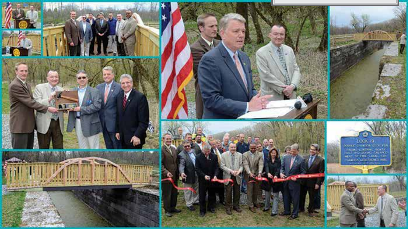
This collage of photos was produced to commemorate the 2012-'13 renovation and bridge construction project that saved Historic Lock 19 and was recognized with a major collaborative volunteerism award. Photo courtesy of www.DaveFeiden.com .
