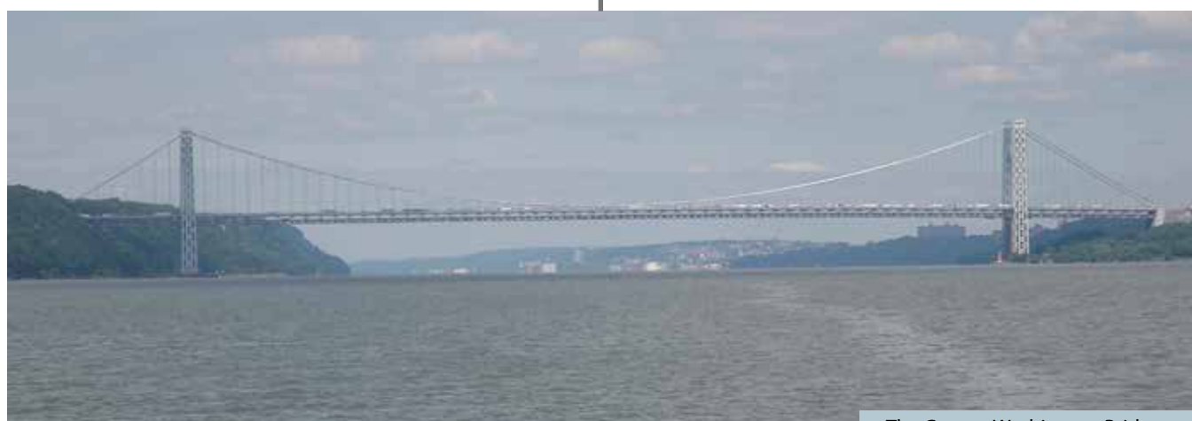
The George Washington Bridge.
